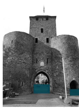
Floodgates The old town of Ahrweiler is surrounded by thick wall and a trench inside. This area contains the traditional Timber houses which are located densely. In this area, a common measure such as use of Floodgates is preferable instead of individual flood proofing of each building.
