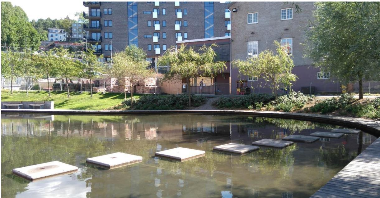
**Figure 2.2(B)** – Kværnerdammen is located on the Alna water course, at a former industrial site. The pond basin is concrete, without emergent vegetation. It is vacuumed to remove algal growth. (Photo: July 2017)
