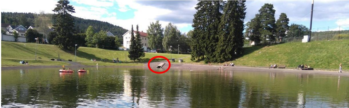
**Figure 2.2(A)** – Årvoll badedam (B12) is located on Hovinbekken stream, and receives water flowing from Årvoll isdam (E04). The inflow pipe is circled in red. The pond basin is asphalt and there is no emergent vegetation.
