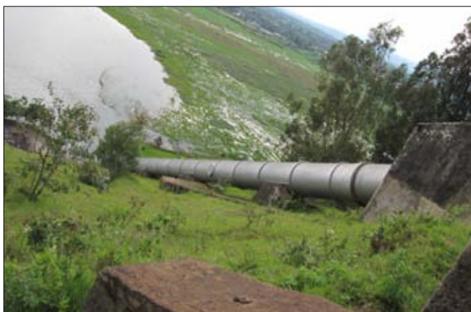
The vertical drop between Lake Burera and Lake Ruhondo is used to generate hydro-power. Water is directed using this pipe. Eugene Apindi Ochieng
