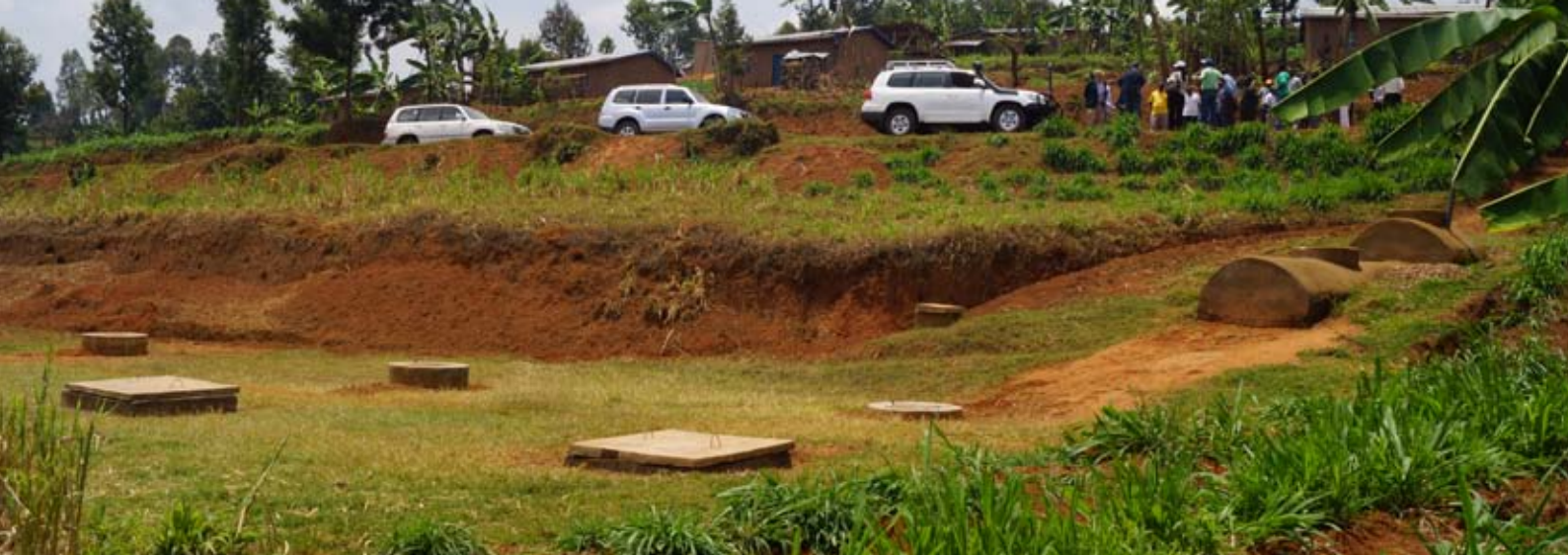
Muyebe green village rainwater harvesting underground storage manholes
